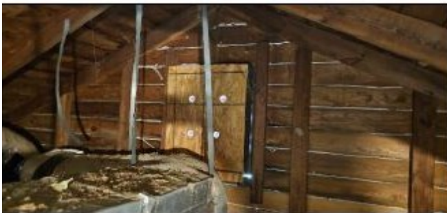
37. Gable vent covered with plywood
