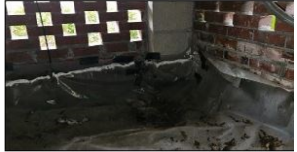
69. Crawlspace below grade
