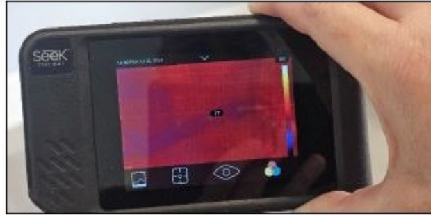
34. Moisture at baseboards
