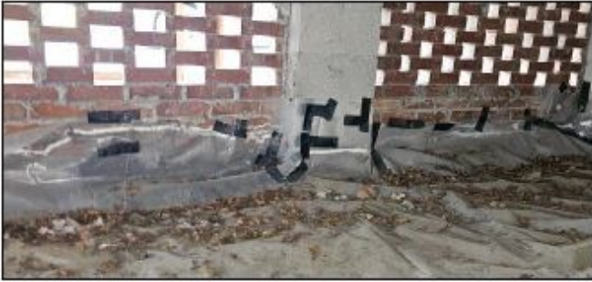
68. Vapor barrier "taped" to wall
