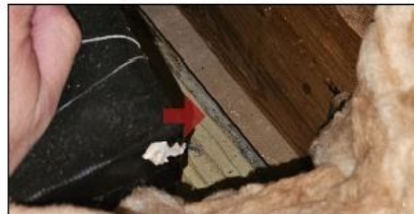
46. Edge of drywall visible from the attic
