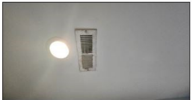
24. Visible growth on register
