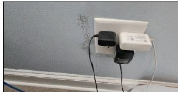
8. Visible growth around outlet
