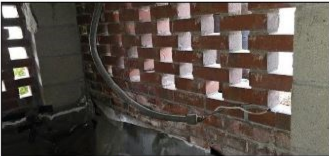
70. Crawlspace below grade
