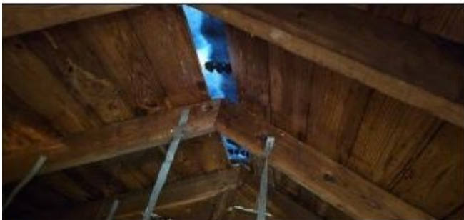
39. Ridge vent looks adequate
